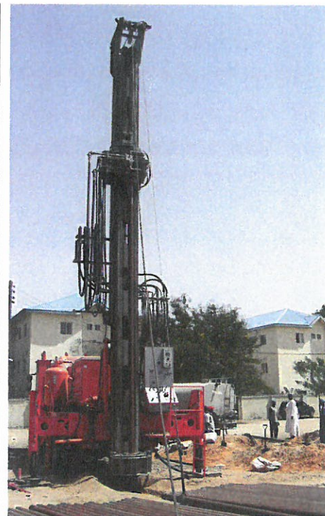
The Watertec 40 rig is drilling boreholes to increase water supply at various locations in the Nigerian state of Borno. Photo by Dando Drilling International
